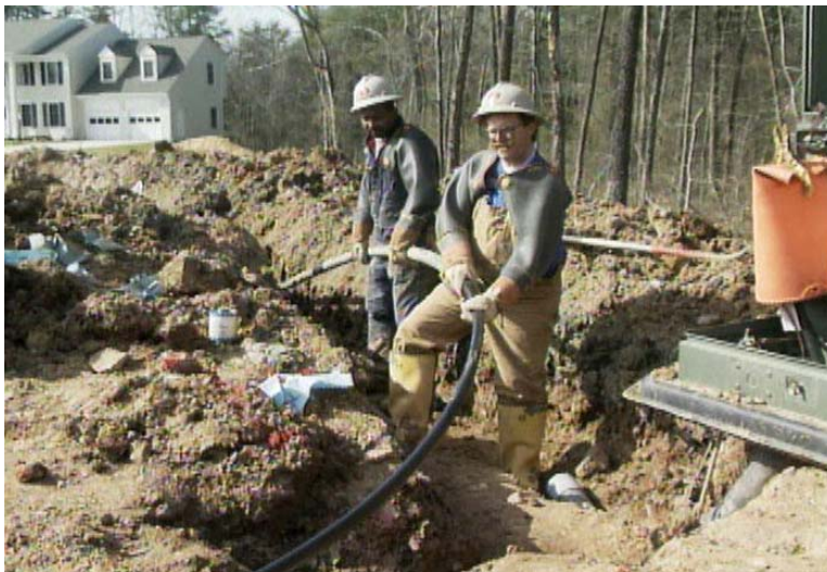
Figure 13: Placing Underground Distribution Cable in an Open Trench
