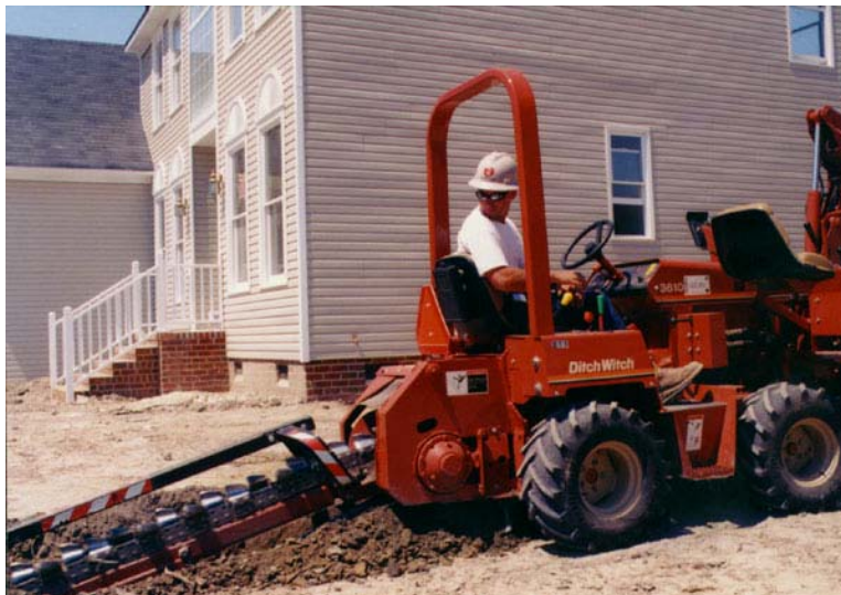
Figure 11: Typical Trenching Operation for Residential Services
