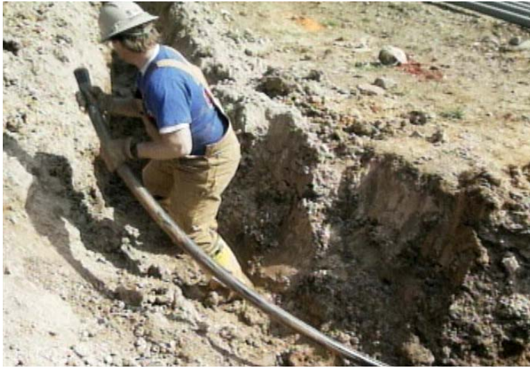
Figure 12: Installing Flexible Conduit in an Open Trench
